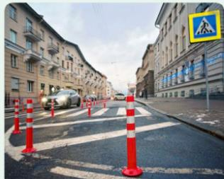
Transverse Striping and Flex-Post/Bollard Curb Extensions
