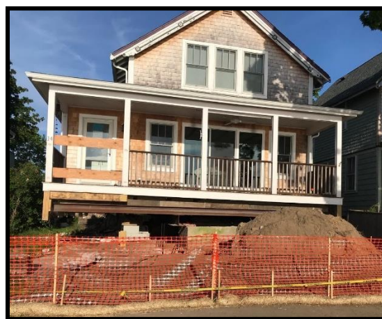
Figure 4-56 Edwin Street Elevation Project A FEMA hazard mitigation grant helped a resident elevate their Edwin Street home (photo credit: Barrington Patch)
