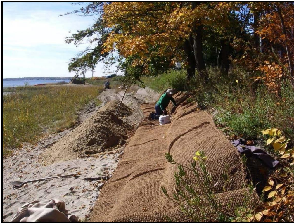
Figure 4-57 Bank regrading at Allin's Cove (photo credit: Save The Bay)
